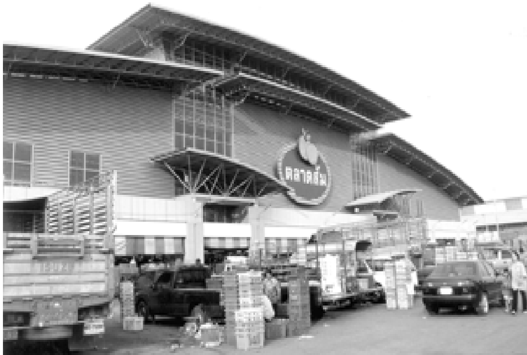
Without careful control congestion may prevent access to market buildings - Agricultural Market of Thailand
